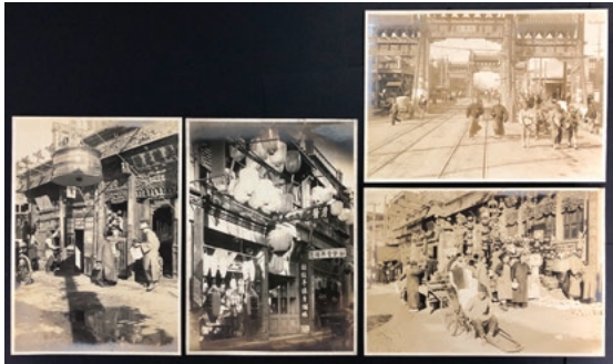
2301 1930s four old photos of Beijing Dashilan and Archway. They are in good condition. Size: 11 x 15cm 1930年代北京大柵欄及牌樓老照片4枚。保存狀態良好。
