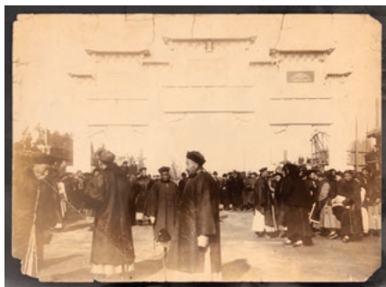
2278 1903 an old albumen print photo of Completion ceremony of the Clemens von Ketteler Memorial Stone Arch in Beijing. There are several small cracks on the top. Size: 15 x 21cm 1903年北京克林德男爵紀念石碑坊落成禮蛋白照片。頂部有數處小裂·品相中上
