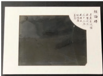
2249 1870-1890s rare large glass negatives of Zhen Hai Lou building in Guangzhou province, with a crack on the right from top to bottom, with a photocopy print from the glass negatives. Size: 16 x 21cm 1870-1890年代廣州省城鎮海樓珍罕大型玻璃底片·右邊有一度由上至下的破裂·附該玻璃底片的影印本一頁。
