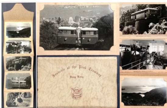
2397 1940s a souvenir of the Peak Tramway Hong Kong. With five real photos, including looking from the top to Cheung Chau, the engine room, car crossing peak viaduct, cars at crossing point and the beginning of the ascent. Excellent appearance, highly collectible.
