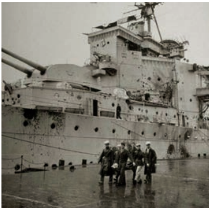
A much-battered H.M.S. London on reaching port.
